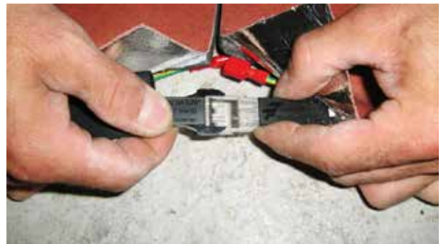
MODULE CONNECTION USING IP67 CONNECTORS
