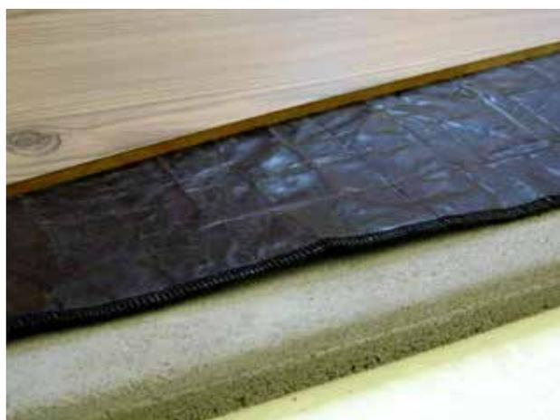
PANEL BETWEEN CONCRETE SCREED AND WOODEN FLOATING FLOOR
